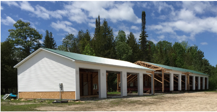
Pole barn being dismantled and moved.
